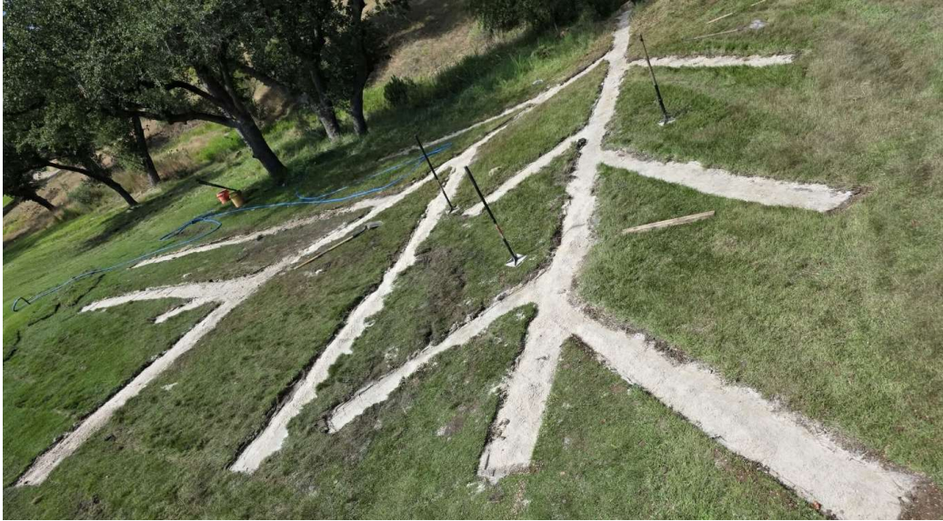
Green #16: Completed Drainage Trenches
