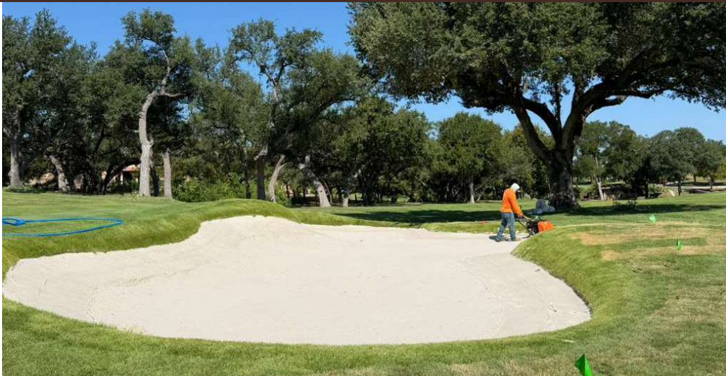
Green #10: Bunker Sand Installation and Final Grading
