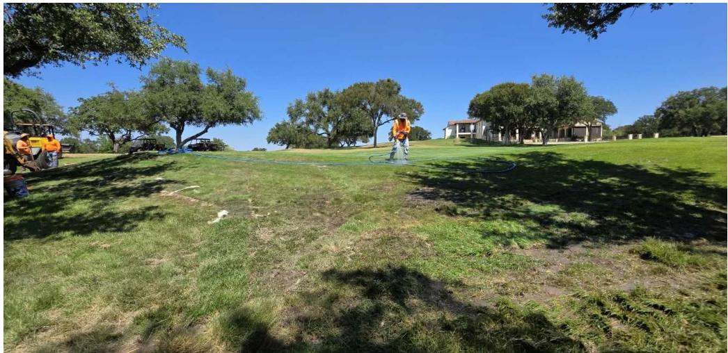
Green #16: French Drain Excavation and Installation
