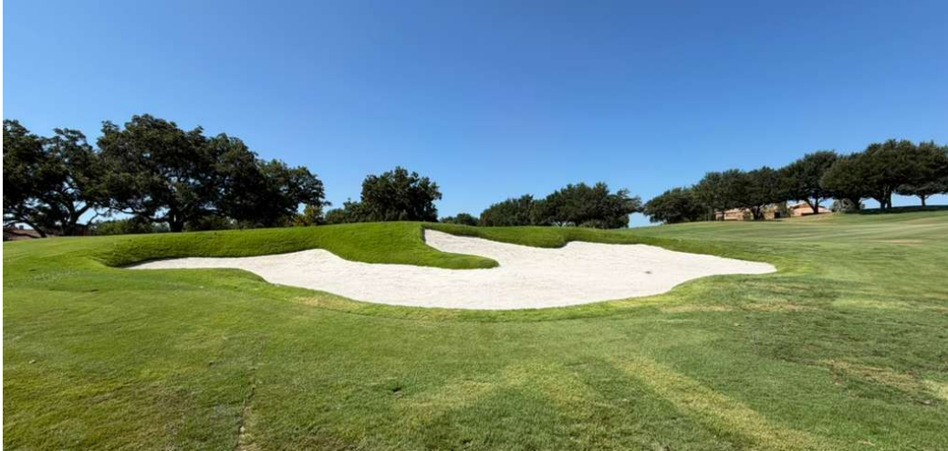
Green #9: Bunker Sand Installation and Final Grading
