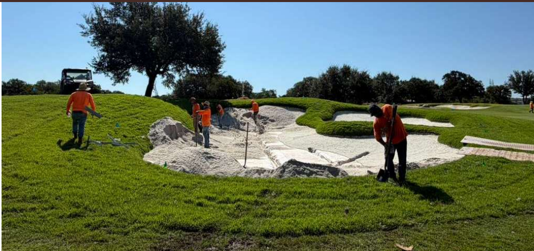
Green #13: Fairway Bunker Sand Installation
