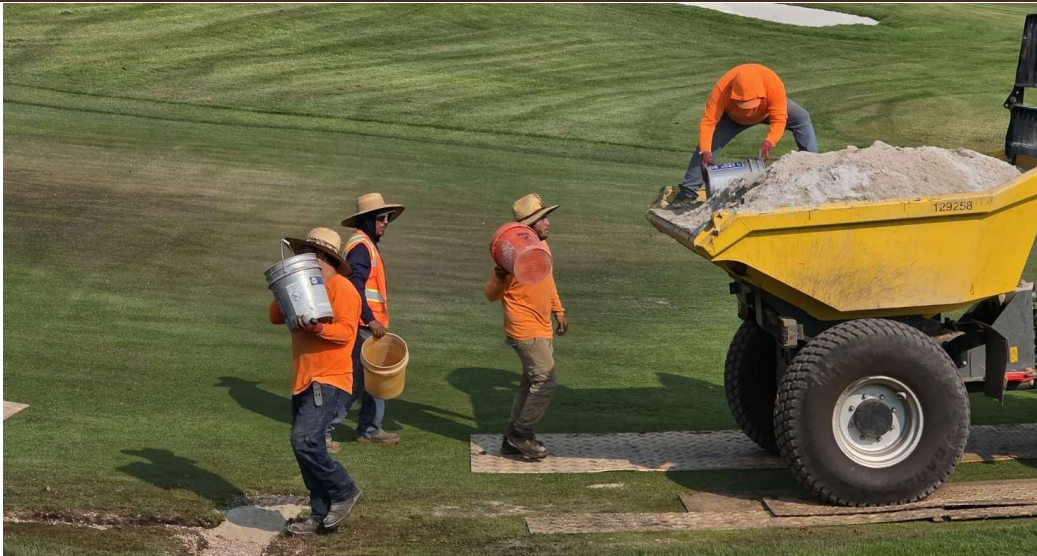
Green #9: Gravel and Sand Backfill for French Drain
