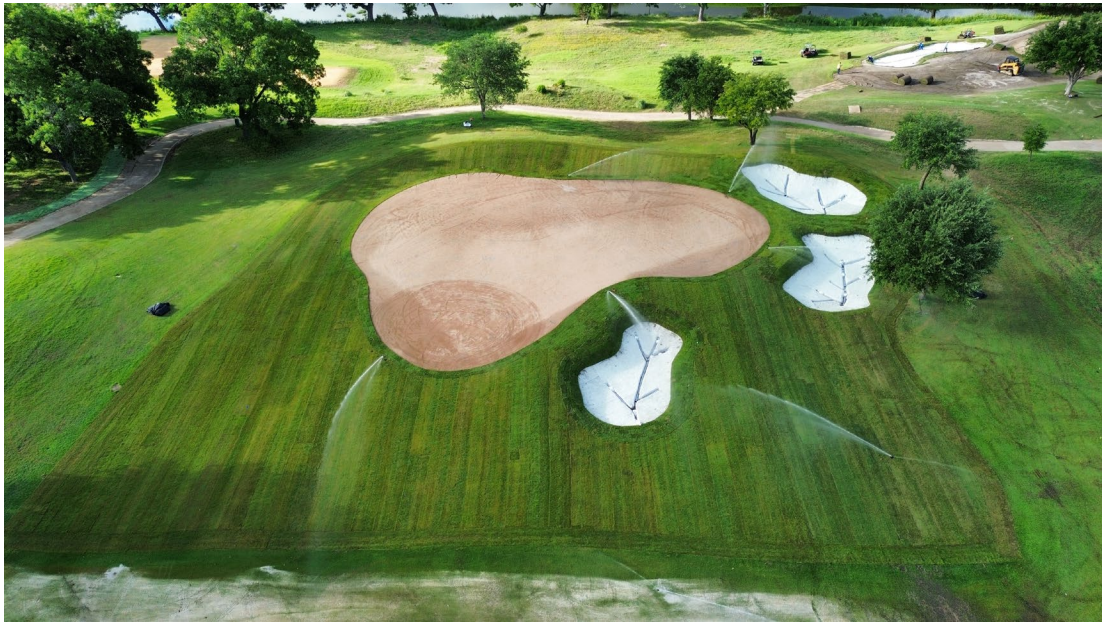
Hole #2 Collar & Approach Sod Installation — June 13, 2026
