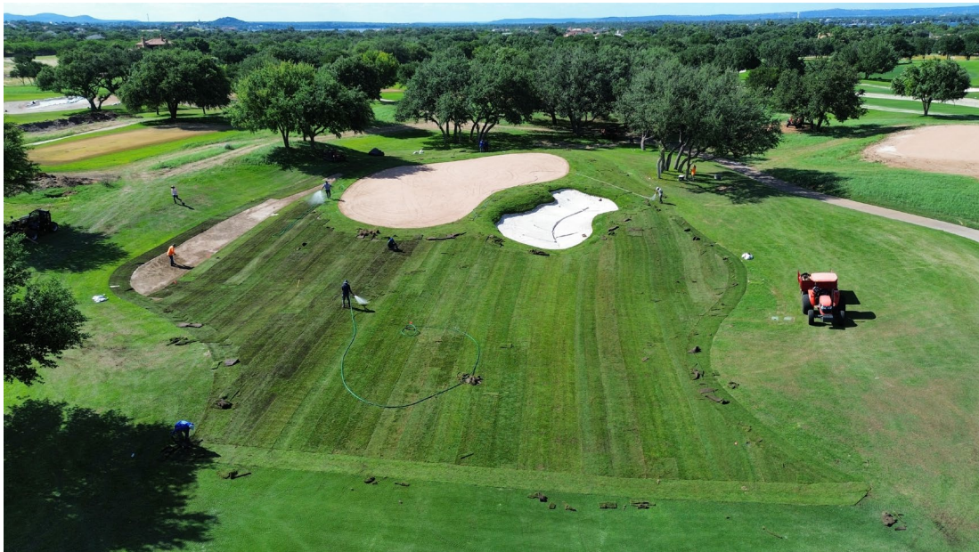
Hole #1 Collar & Approach Sod Installation — June 13, 2026
